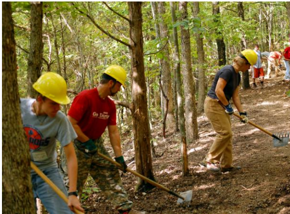
Members of Crew 5 work to clear rocks and create the tread (trail surface) using McLeods: a tool that combines a rake and hoe in one
