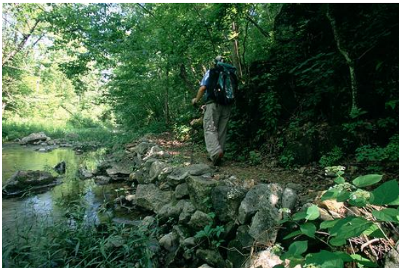
This photo, included in the proposal supporting the OT’s nomination for NRT designation, shows a rock retaining wall built on Neals Creek which allows the Middle Fork section to pass along a bluff
