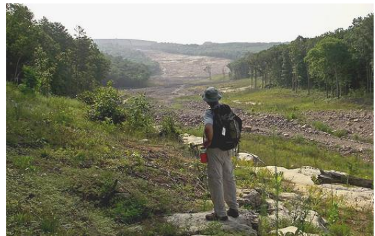
The scour valley and rhyolite rubble caused by the Taum Sauk reservoir breach
